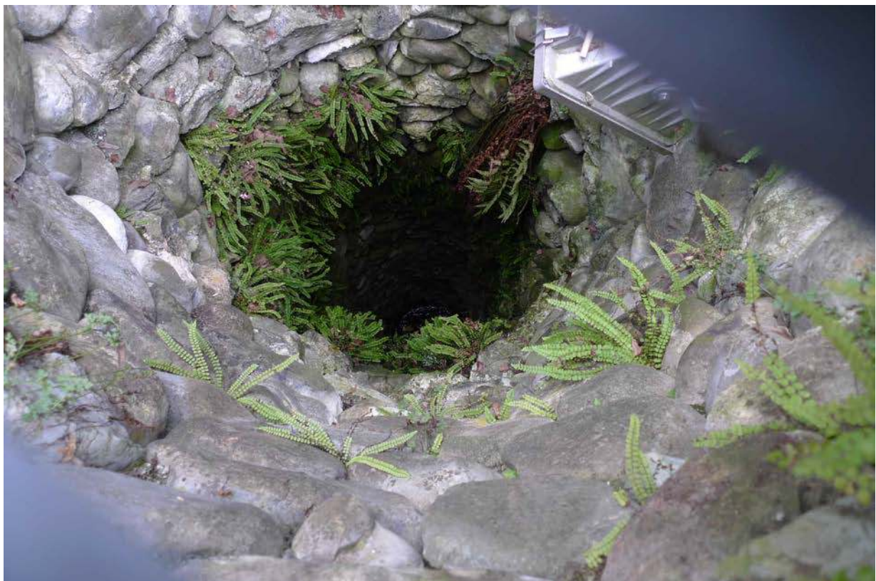
Blick in den Brunnenschacht (2016)
